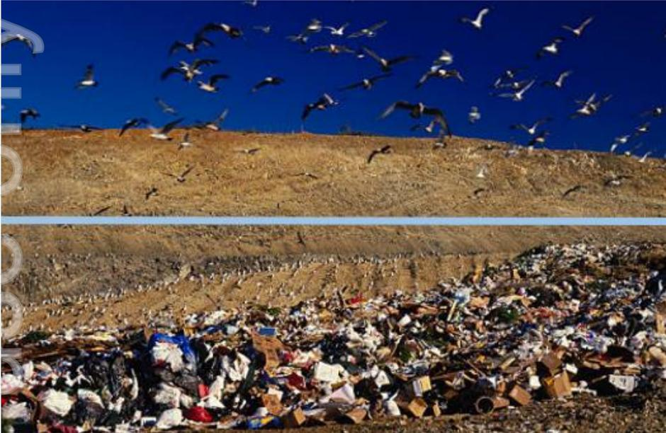
The blue highlight line indicates where an active manufactured zeolite layer could function to intercept and destroy methane emitted from the underlying refuse.
